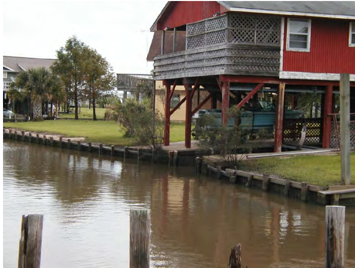
Typical Class 4 BH2—6" to 10" Pilings, 2" Treated Lumber
