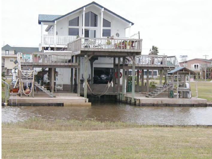
Typical Class 4 BH2—6" to 10" Pilings, 2" Treated Lumber
