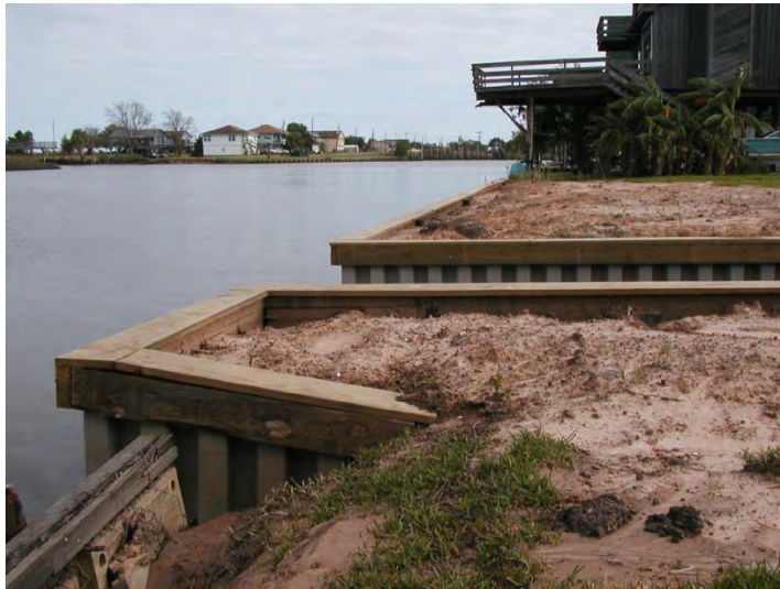
BH2—Class 5 Synthetic Material in Excellent Condition.
